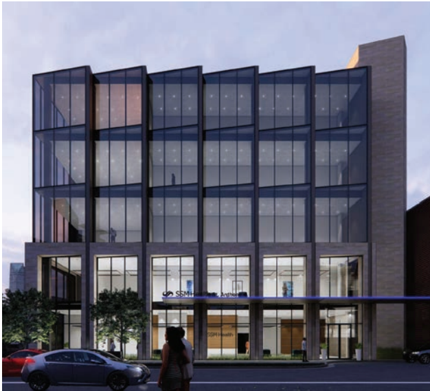
Artist rendering of the to-be-named SSM Health St. Anthony building to house a Comprehensive Digestive Disease Center, Advanced Endoscopy Center and surgery services.
